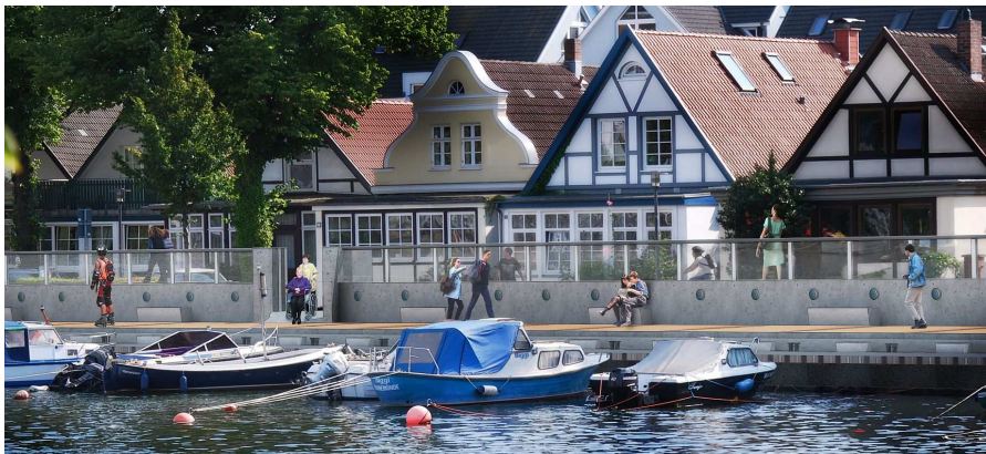
Figure 2: Future view from the river Alter Strom to the storm flood protection wall [2]
